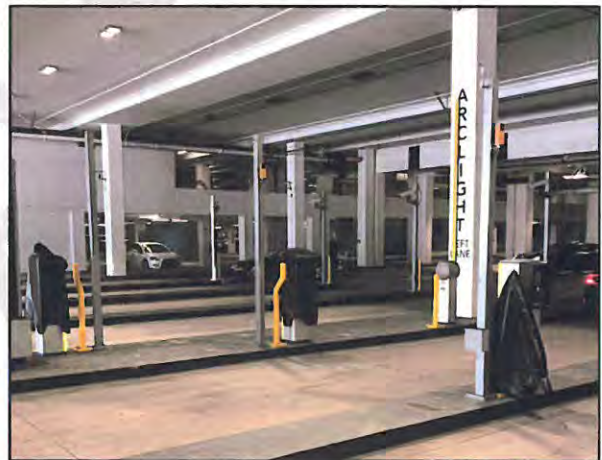
Image 24. SKIDATA PARCS gated entrance with LPR at UTC Garage in San Diego
