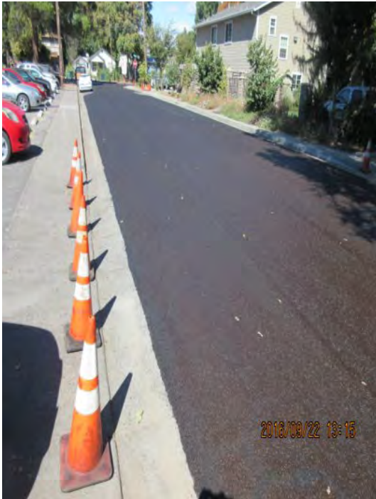
ROADWAY AFTER SLURRY SEAL
