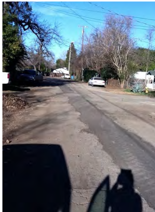
ROADWAY WITHOUT SLURRY SEAL
