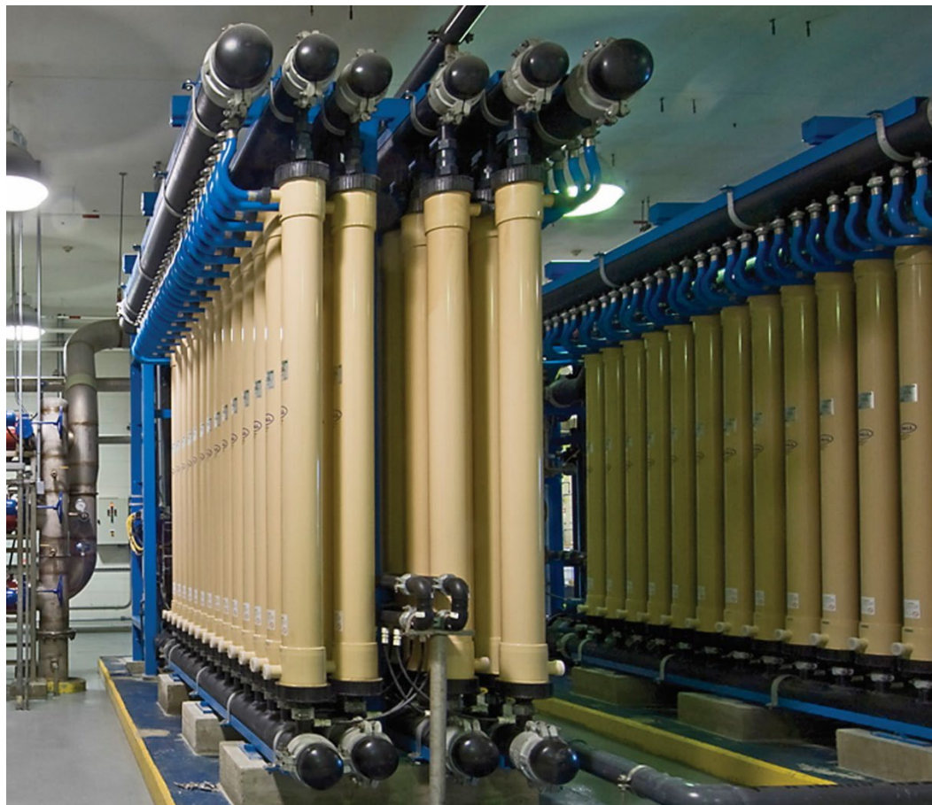
Figure 8.4 Example Installation of Pressurized UF Membranes
