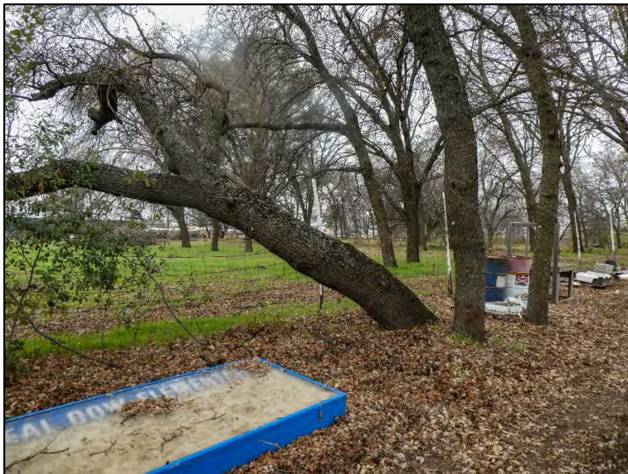
Tree #53 is arching majorly onto the neighboring lot to the west. Photo Date 01-20-20.
