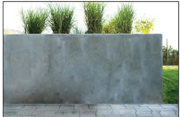
SMOOTH CONCRETE WALL EXAMPLE
