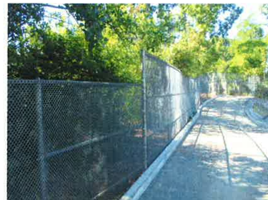
6' TO 8" CHAIN LINK FENCE TRANSITION
