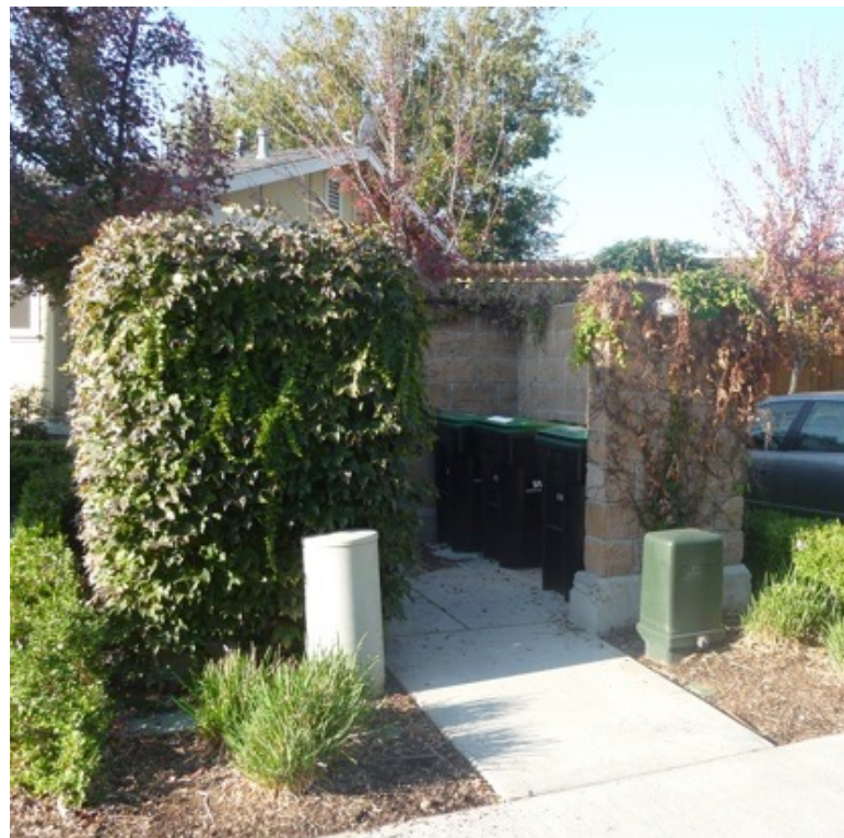
TRASH ENCLOSURE 6' tall concrete block wall trash enclosure landscaped with lilac vine.
