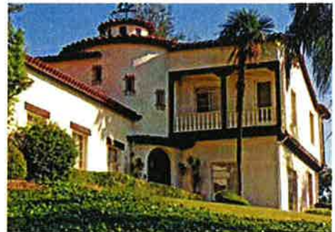
Bridgford House (1927) 401 Cannon Lane
