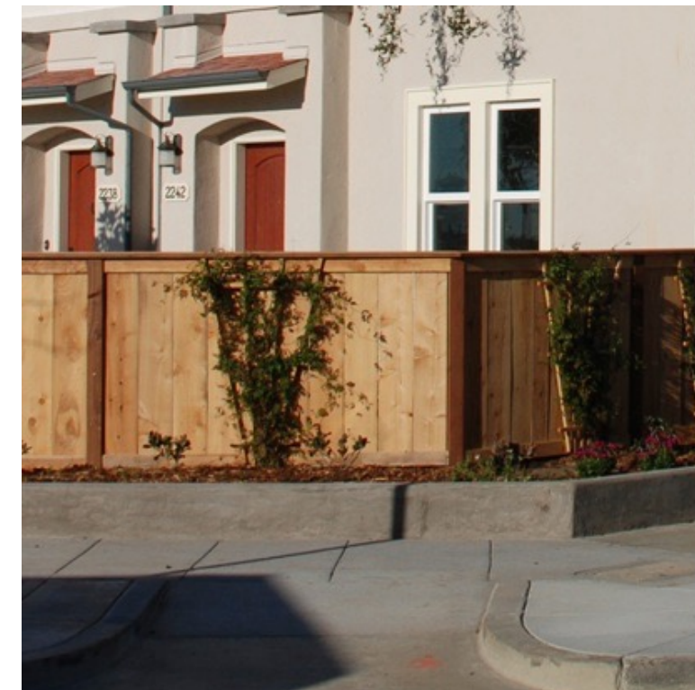
FENCE (Typical) 4' & 6' tall wooden fence with beveled cap and trim boards at top and bottom.
