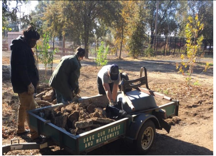
Figure 2: Comanche Creek cement removal
