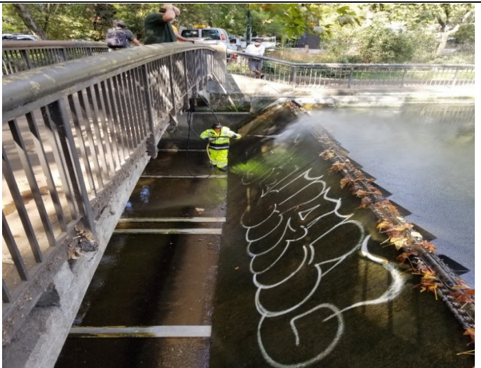
Figure 5: 1 Mile Dam graffiti removal
