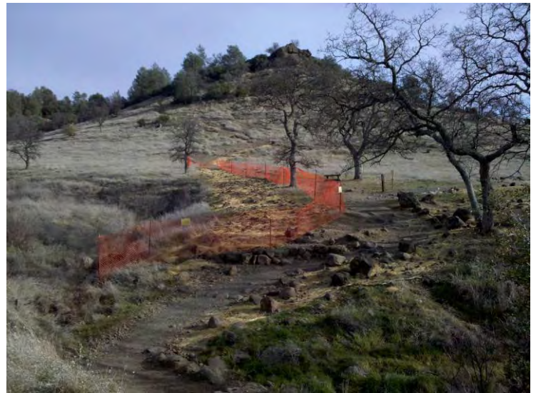
2. Improved crossing and Middle trail work.
