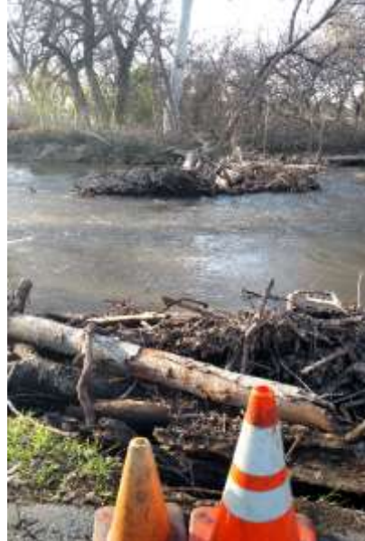
High water flows thru the log jam area. Wood debris was moved closer to the bank to offer roughness and mild bank protection.
