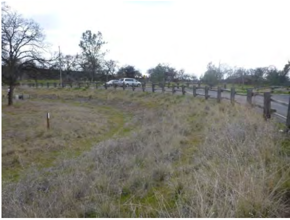
Photo 1: Eastern slope of landfill area overview. Vegetation is in great condition and there's no evidence of erosion.
