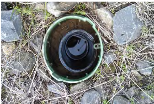
Photo 3: Monitoring sump with cap removed (depth to water approximately 18 inches).
