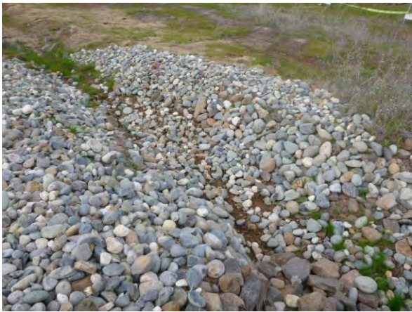
Photo 3: New cobbles near northernmost culvert.
