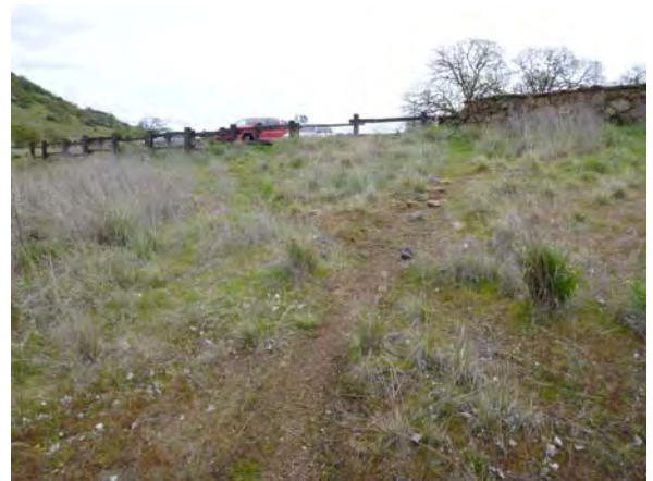
Photo 4: Established pirate trails down northwest-facing slope of containment cell, below parking lot.
