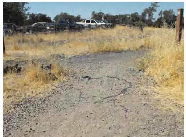
Photo 4: Sections of geotextile mat or weed barrier cloth is exposed near monument 2.
