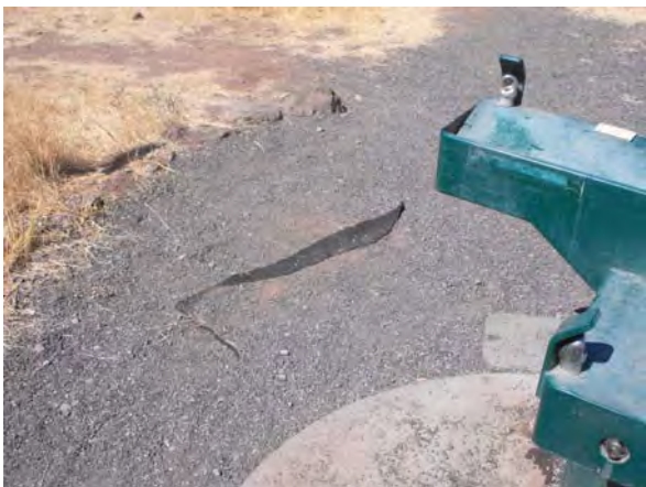
Photo 3: Either geotextile matting or weed barrier cloth is exposed on a southwest path next to the drinking fountain.
