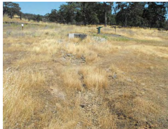
Photo 6: Channel from the west side culvert which may be vulnerable to increased erosion
