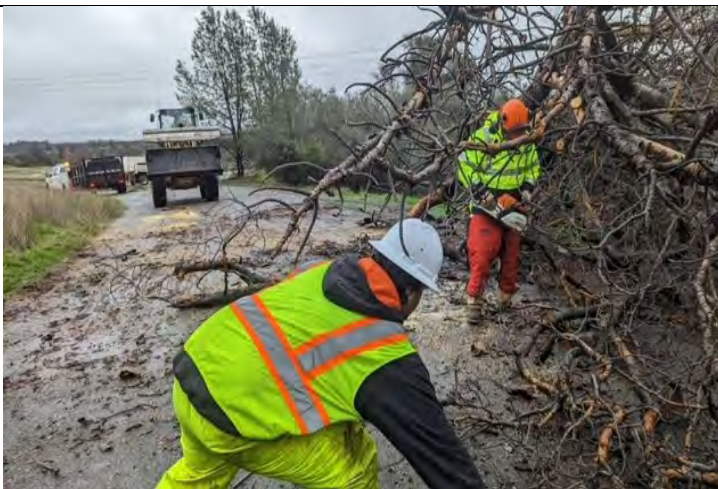
Figure 5 Five Mile down tree
