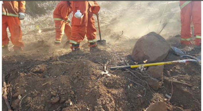
Crew preparing to install a straw bale dam.
