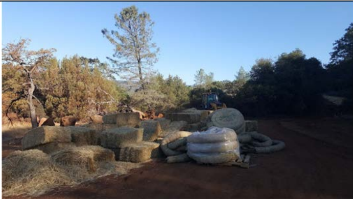
Staging area with straw, wattles, stakes, and jute.
