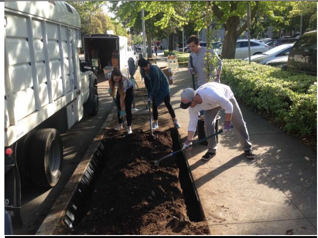
Installing root barriers.
