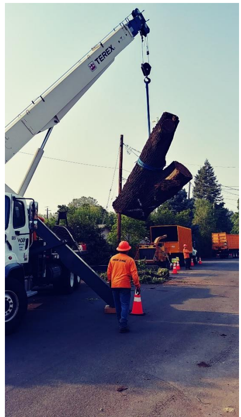
Figure 3, right. Contractor removes large dying Black walnut on 16 th St.
