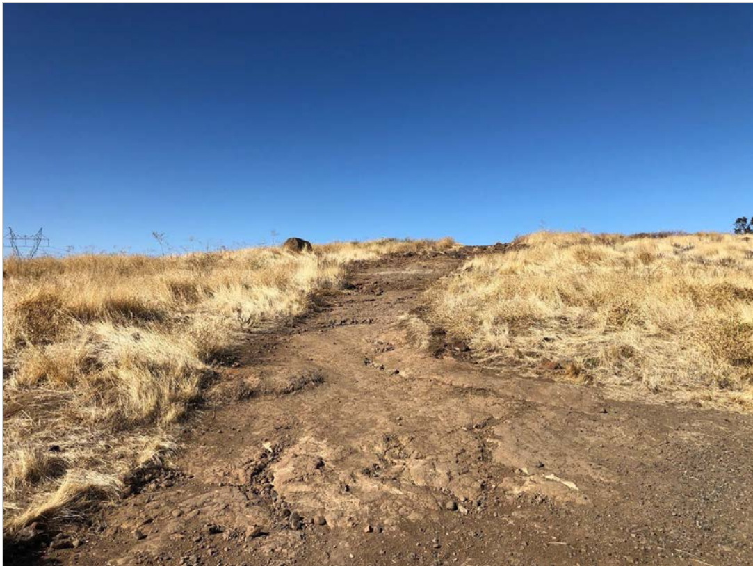
Figure 3: Rocky Conditions, Shallow Soil, and Severe Erosion of North Rim Trail in Upper Bidwell Park, Chico CA.
