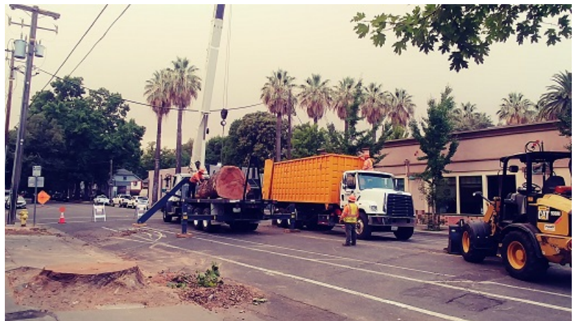
Figure 4 WCA removing 80' Eastern sycamore. 5 th and Ivy. Log removal for transportation to WCA sawmill.
