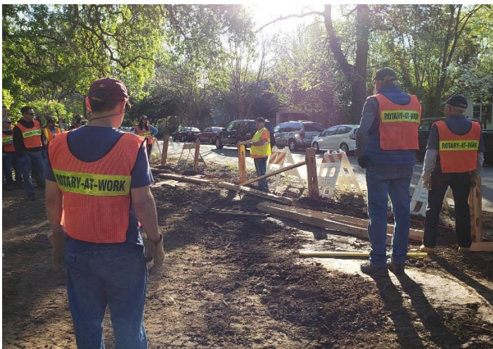
Figure 3 - Noon Rotary installs split rail fencing
