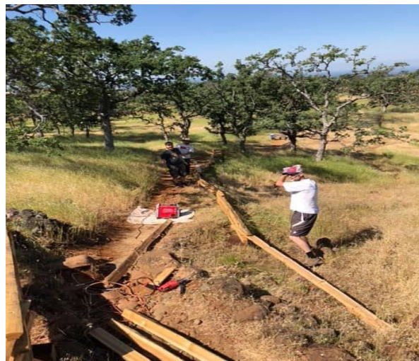
Figure 6 – Staff and ORAI install split rail at PPDG
