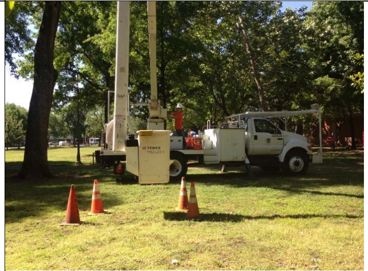
Figure 4 Employees had to safely operate the ground controls on the bucket truck and position it in a designated coned area
