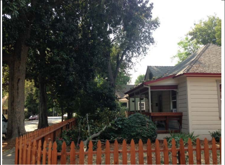
Figure 2. Response to limb that hit house at 494 E 7th St 9-5-17.
