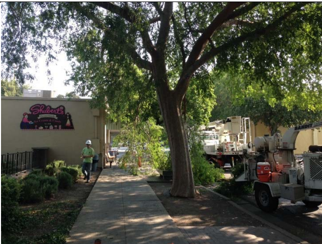
Figure 7. Response to broken limbs in Elm tree at Shubert's ice cream on E 7 th St 9-5-17.
