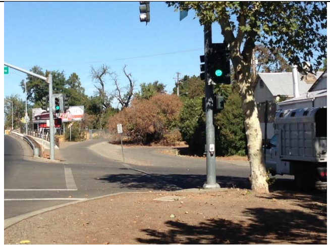
Figure 3 After pruning for signal visibility
