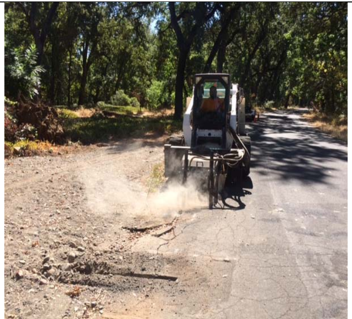
Figure 4 ROW crews repair Petersen Drive
