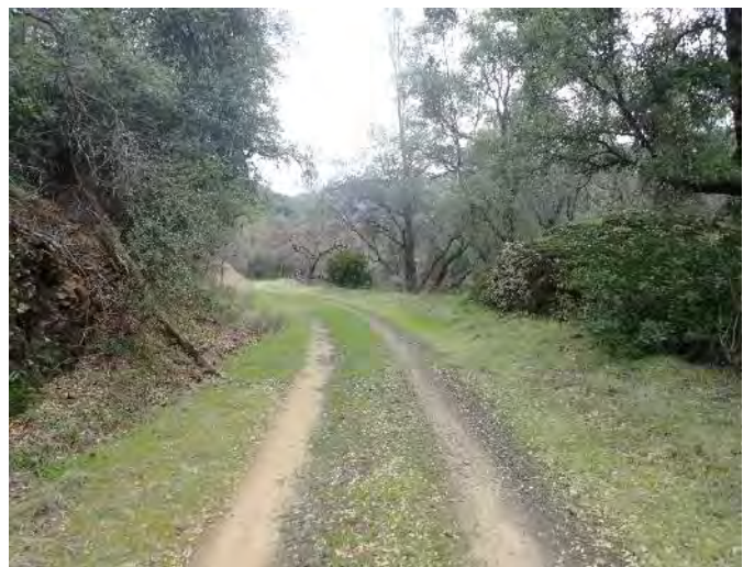
Figure 5. The bare surface area on the road is reduced beyond the gate located at the Diversion Dam Parking Area. Reduced levels of vehicular use can allow vegetation to cover the road and reduce the intensity and magnitude of road-related runoff, erosion and sediment delivery.
