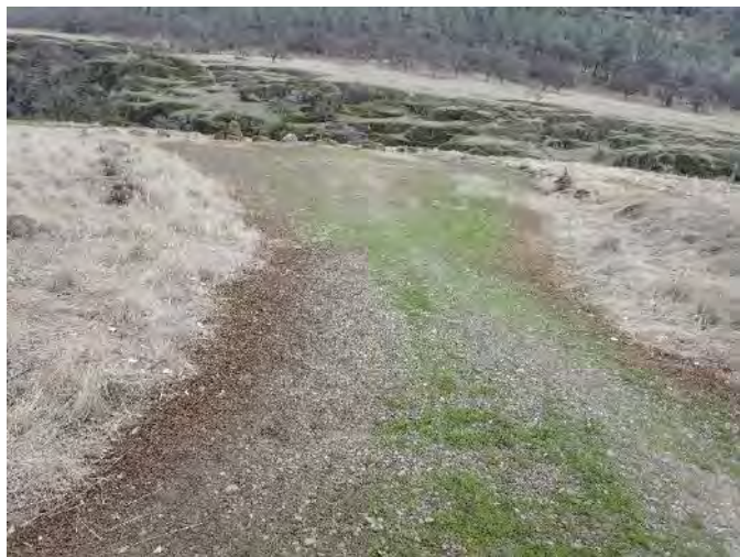
Figure 4. Each individual parking areas showed minimal signs of erosion or sediment delivery. It will important to reduce any potential run-on that may negatively affect these parking areas.
