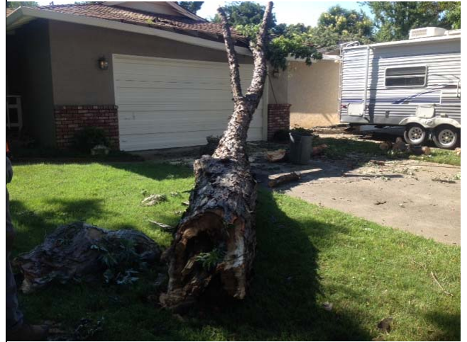
Figure 2. Emergency response to a large broken silver maple limb that hit a house on White Ave. 6-19-17.
