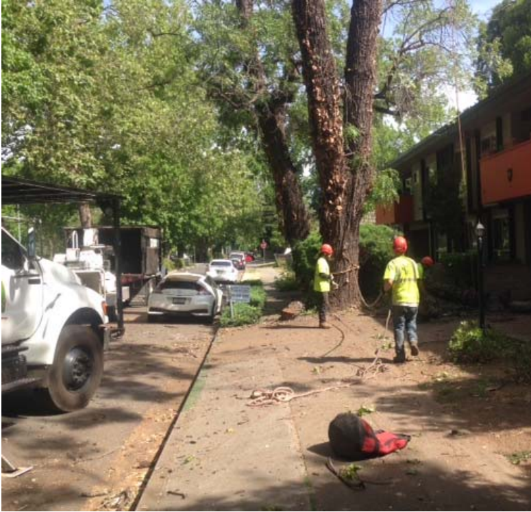
Figure 5. Twin Cites Tree Service setting up rigging lines for the removal 6-5-17.
