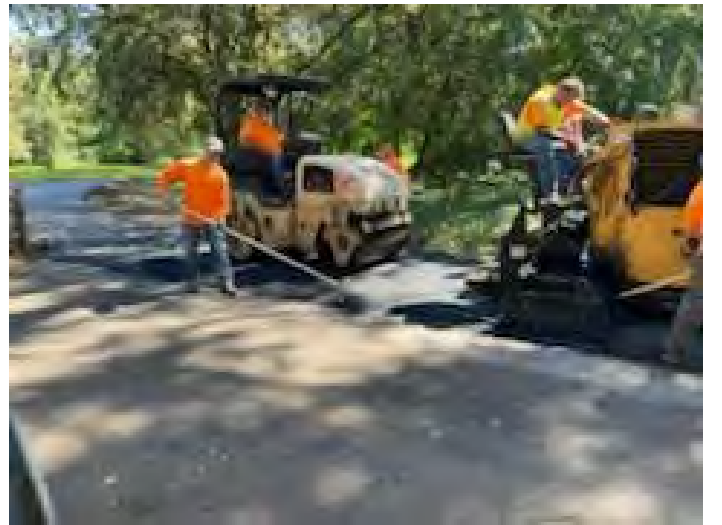
Figure 4-Repaving the bike path
