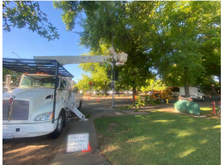
Figure 2 Tree Division crew. Maintenance of trees in the ROW
