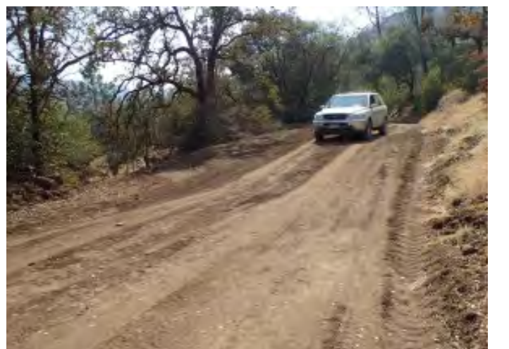
Figure 6- One of 47 rolling dips installed
