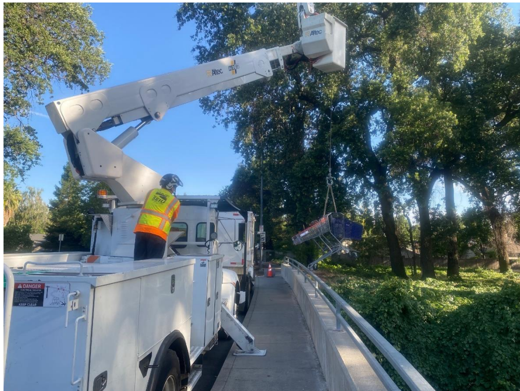
Figure 5 and 6. 6/14/22. Public Works staff. Lindo channel cleanup.
