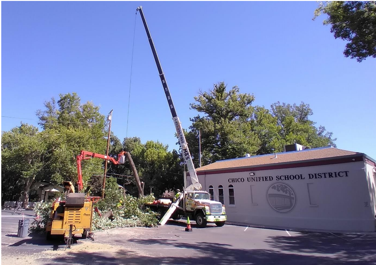
Figure 4. Removal of Linden tree. M&S Wesley emergency contractor.
