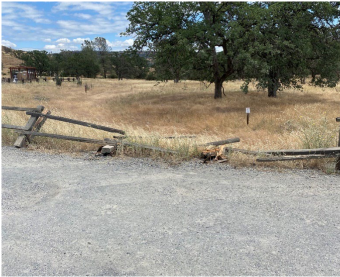
Figure 3 Lot E Split Rail Damage
