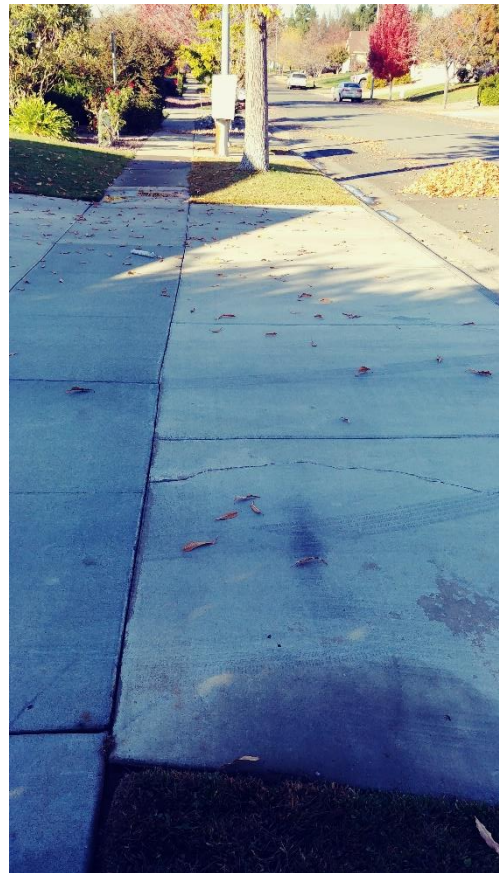
Figure 6. A shallow tree roots in the park strip showing recent mower damage. Figure 7. Driveway and sidewalk. No significant lift. Driveway is cracked but is unlikely to be caused from this tree
