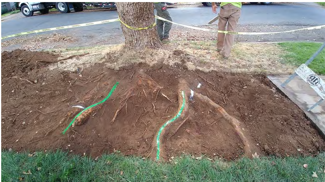
Figure 1. Before and after photographs of sidewalk repair. 945 Alder. Sidewalk was repaired to ADA standards. Most of the roots of the Camphor tree were retained. The bottom photo shows roots marked for shaving.
