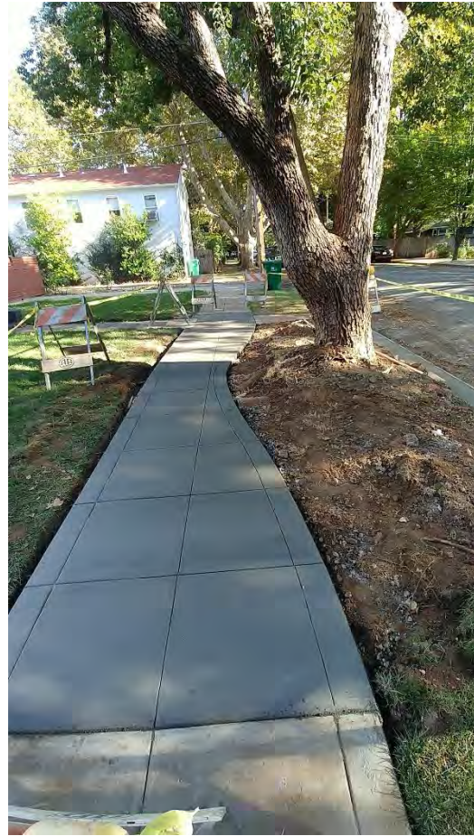
Figure 1. Before and after photographs of sidewalk repair. 945 Alder. Sidewalk was repaired to ADA standards. Most of the roots of the Camphor tree were retained. The bottom photo shows roots marked for shaving.
