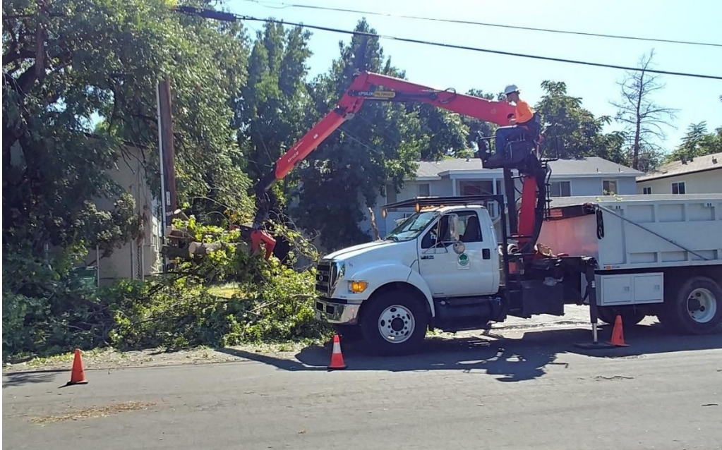
Figure 1. Sweetgum failed during rain event on Klondike ct. public Works responded during emergency hours. Tree Crew later removed debris
