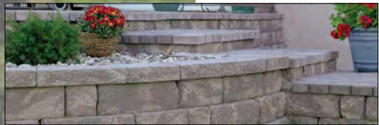
DRY STACK MASONRY WALL
