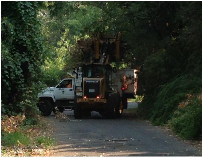
Figure 1. Cleaning up contractor brush piles on South Park Dr. in Bidwell Park
