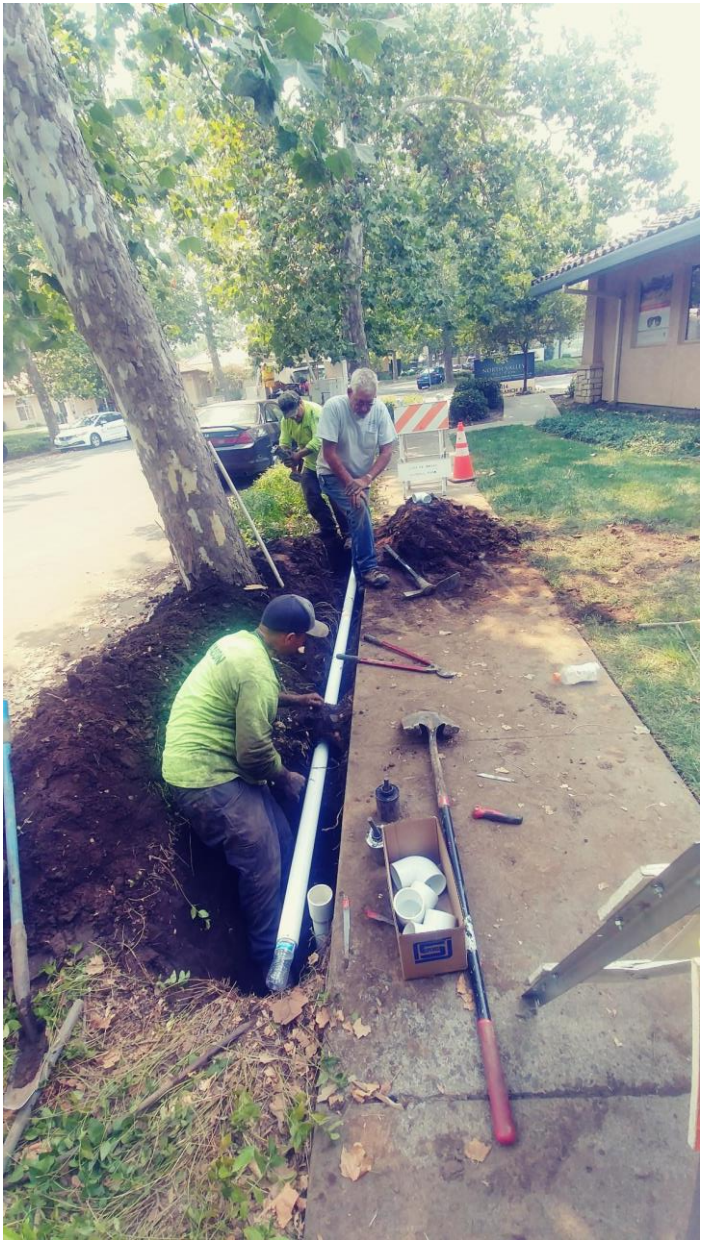
Figure 1 . Dawson landscapes repairing irrigation pipe and preserving tree roots
