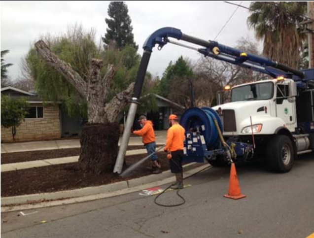
Figure 3. Root excavating training with the right of way department 1-18-18
