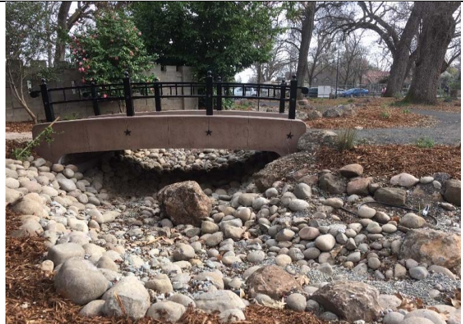
Figure 4 New entrance bridge
