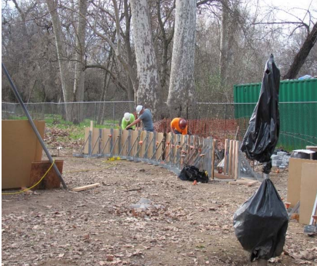
Figure 1 Caper Acre seat wall forming
