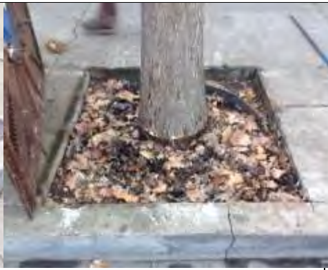
Figure 24. Removing the grate and cage.
