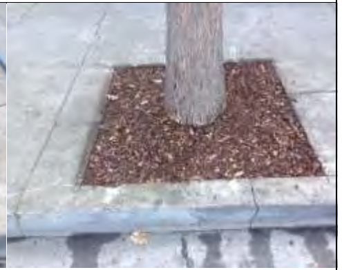
Figure 25. Back filling with mulch will help protect the roots and will make for safe sidewalk traffic.
