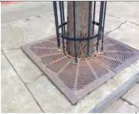
Figure 23. This tree has outgrown the grate and cage and needs to be removed before it causes injury to the tree.
