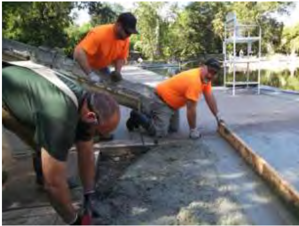
Figure 3. Sycamore pool deck repair.
