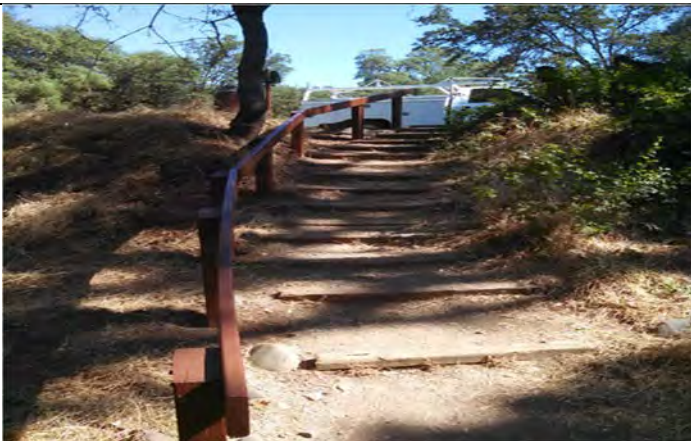
Figure 5: Yahi trailhead staircase
