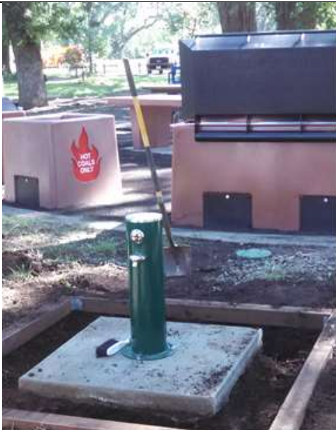
Figure 7 water dispenser ready for cobble.
