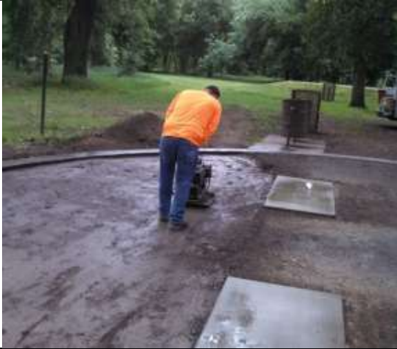
Figure 5 Oak Grove reservation area ready for new fixtures.
