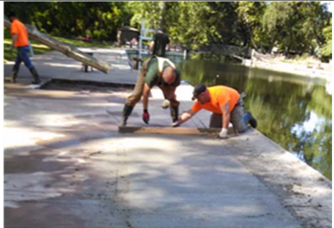
Figure 8. Parks crew continuing repairs to pool deck.
