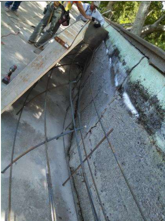
Figure 5. Sycamore pool gets a buttresses to the south wall.
