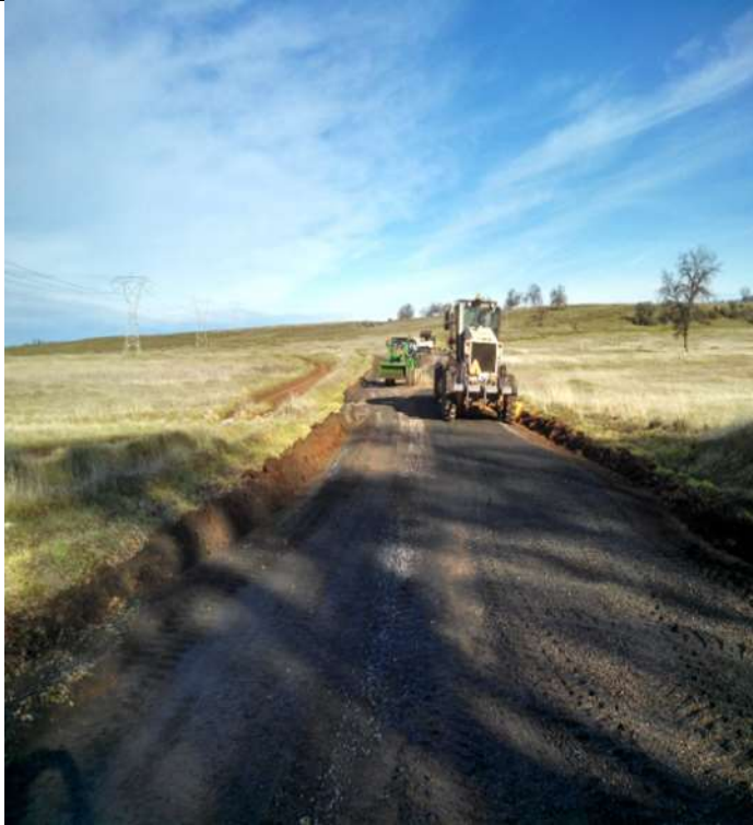
Figure 1. Re-surfacing parking lot B in Middle park.
