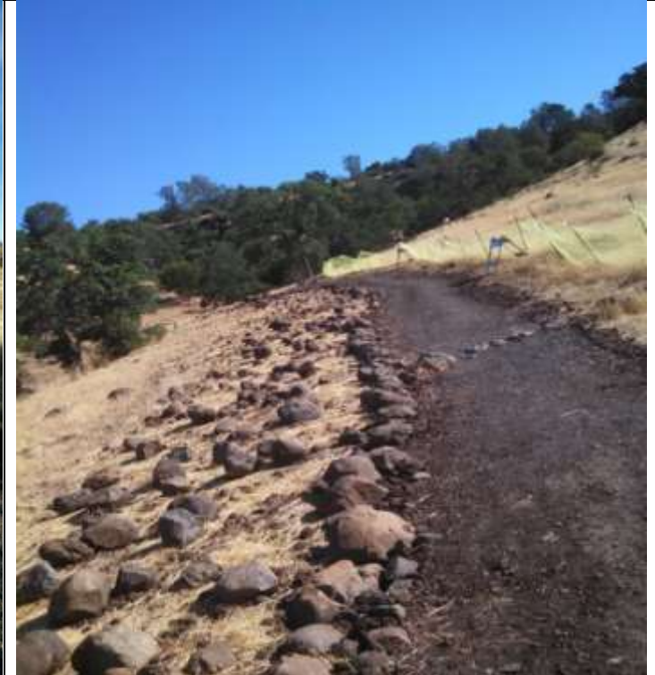
Figure 2. The beginning of Monkey face trail rock work.
