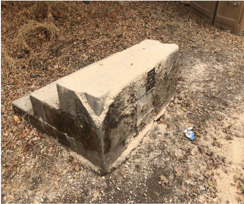
Figure 1: Vandalism to memorial mounting block
