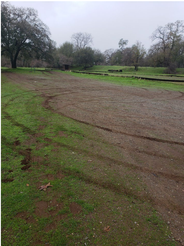
Figure 3: Damage from vehicle "doughnuts"
