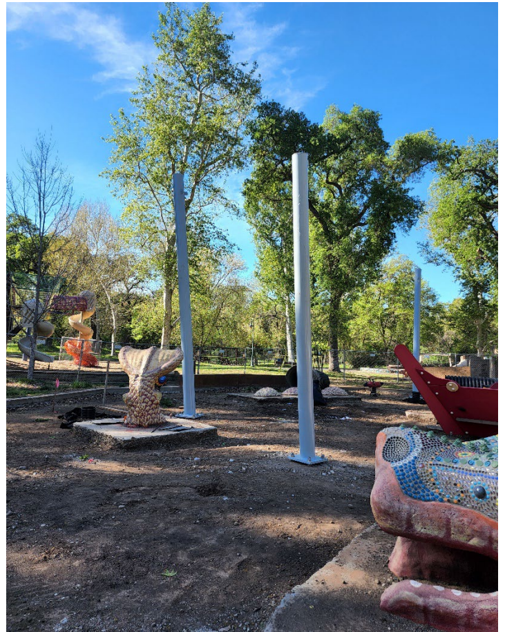
Figure 4: Nico Project Shade Sail Posts
