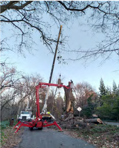
Figure 3 Emergency contractor work on South Park Drive after October storm
