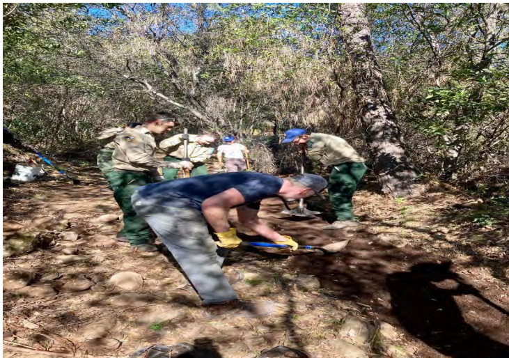
Figure 3: CCC trail repair with Chico Velo
