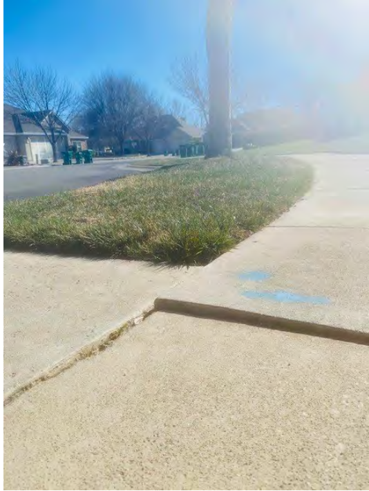
Figure 8 and 9. Slabs lifted by roots. The slab is currently lifted ½”.
