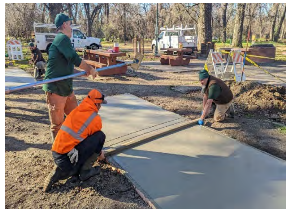
Figure 6: 1- Mile Picnic Area cement pad install
