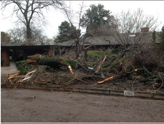
Figure 3. 1351 Woodland Ave large valley oak fell over taking down the power pole and high voltage power lines 1-9-17.
