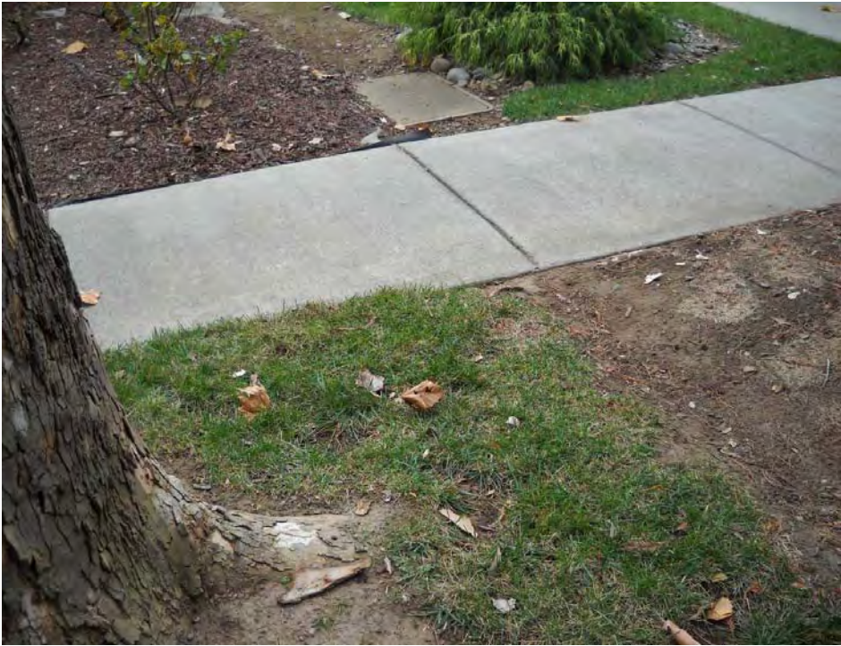
This sycamore tree in the F:1 position has underground utilities a few feet away of the main trunk. They run underground in the dirt area to the gray box labeled PG&E. The utilities in this area consist of phone, cable, gas, and electricity.
