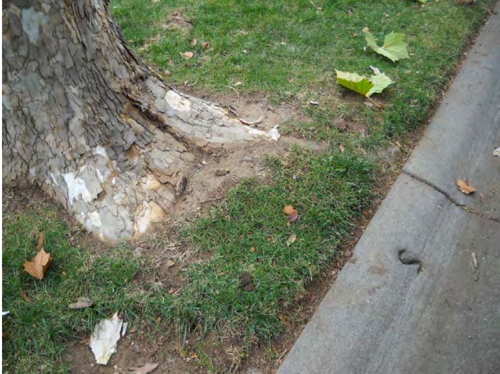
This sycamore in the F:2 position was planted on top of the sewer lateral that runs from the street to the house. The S in the curb stands for “sewer”.
