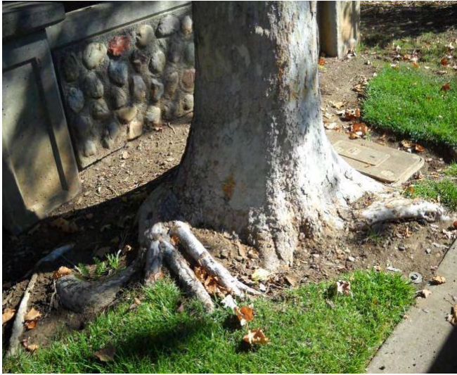
This sycamore tree in the F:1 position is within 12 inches of the water main that supplies water to the 12 units and the residents.
