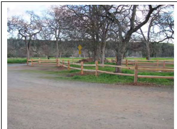
Parking Lot D – split rail installation to protect Blue Oaks.
