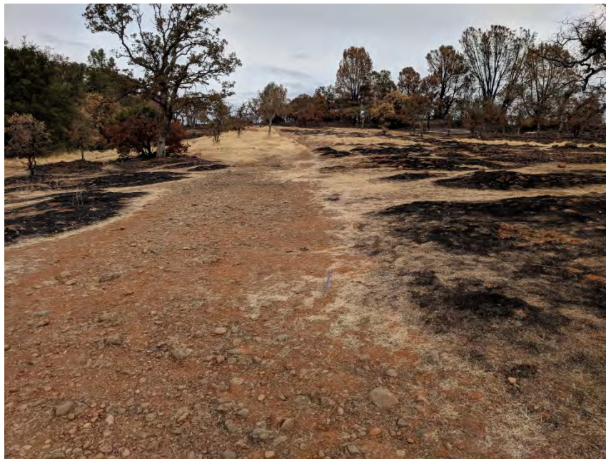
Post fire picture of the disturbed area between tee pad # 14 and 17 looking north
