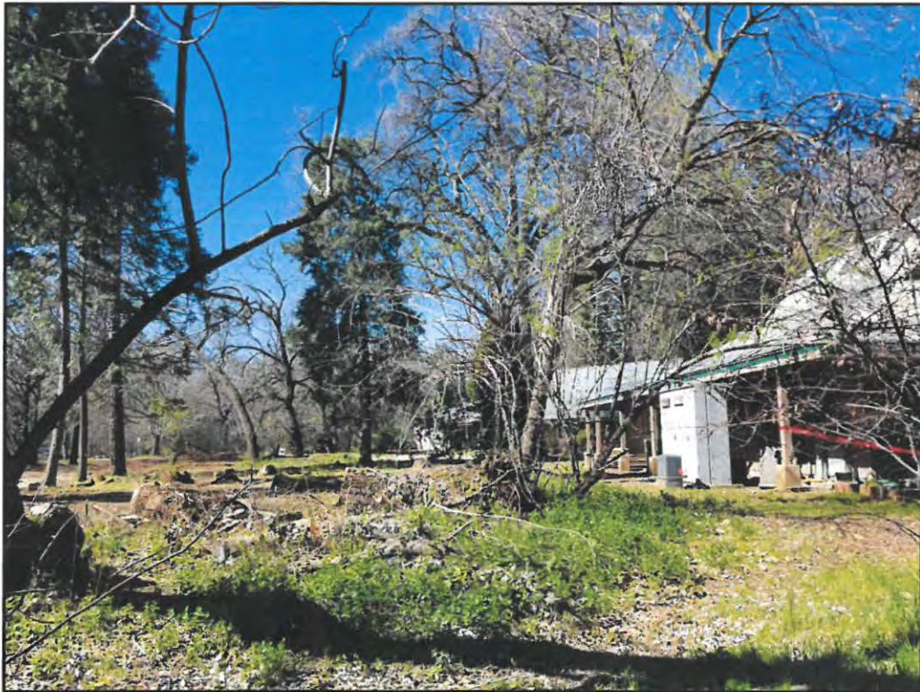
Cluster #4 showed signs of past trimming, but was not impacted by maintenance activities.
