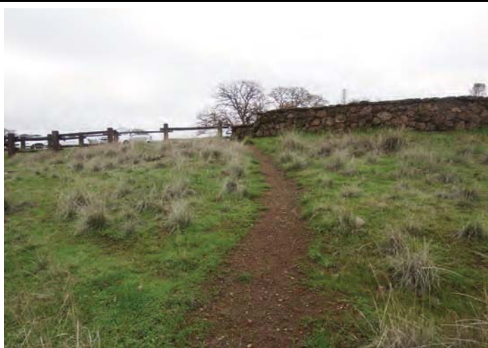
Photo 3: Northwest extent of containment cell (view southeast) Good vegetative cover but unintentional footpath continuing to develop.
