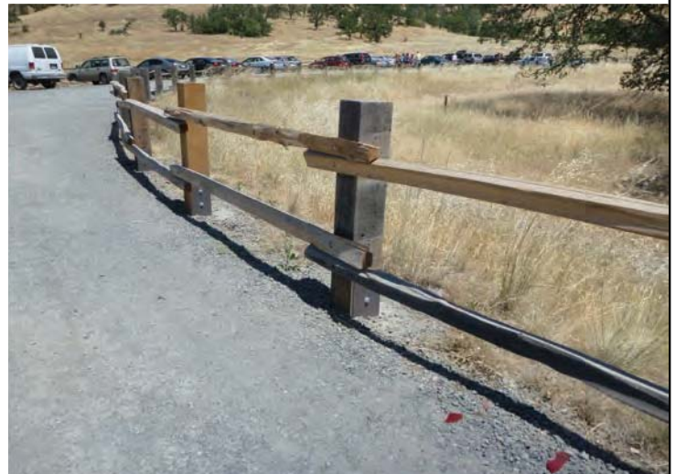
Photo 4: Southern extent of containment cell Note: newly-replaced fence boards (view north)
