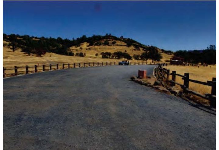
Photo 2: Parking lot area overview (view northeast)
