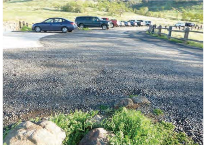
Photo 2: Parking lot area overview (view northeast)
