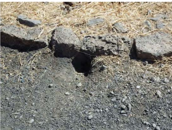
Photo 5: Two rodent burrows were identified on the northern extent to the containment cell
