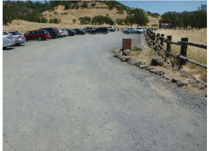
Photo 2: Parking lot area overview (view northeast)
