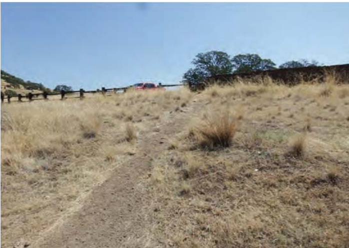
Photo 3: Northwest extent of containment cell (view southeast) Good vegetative cover but unintentional footpaths are developing
