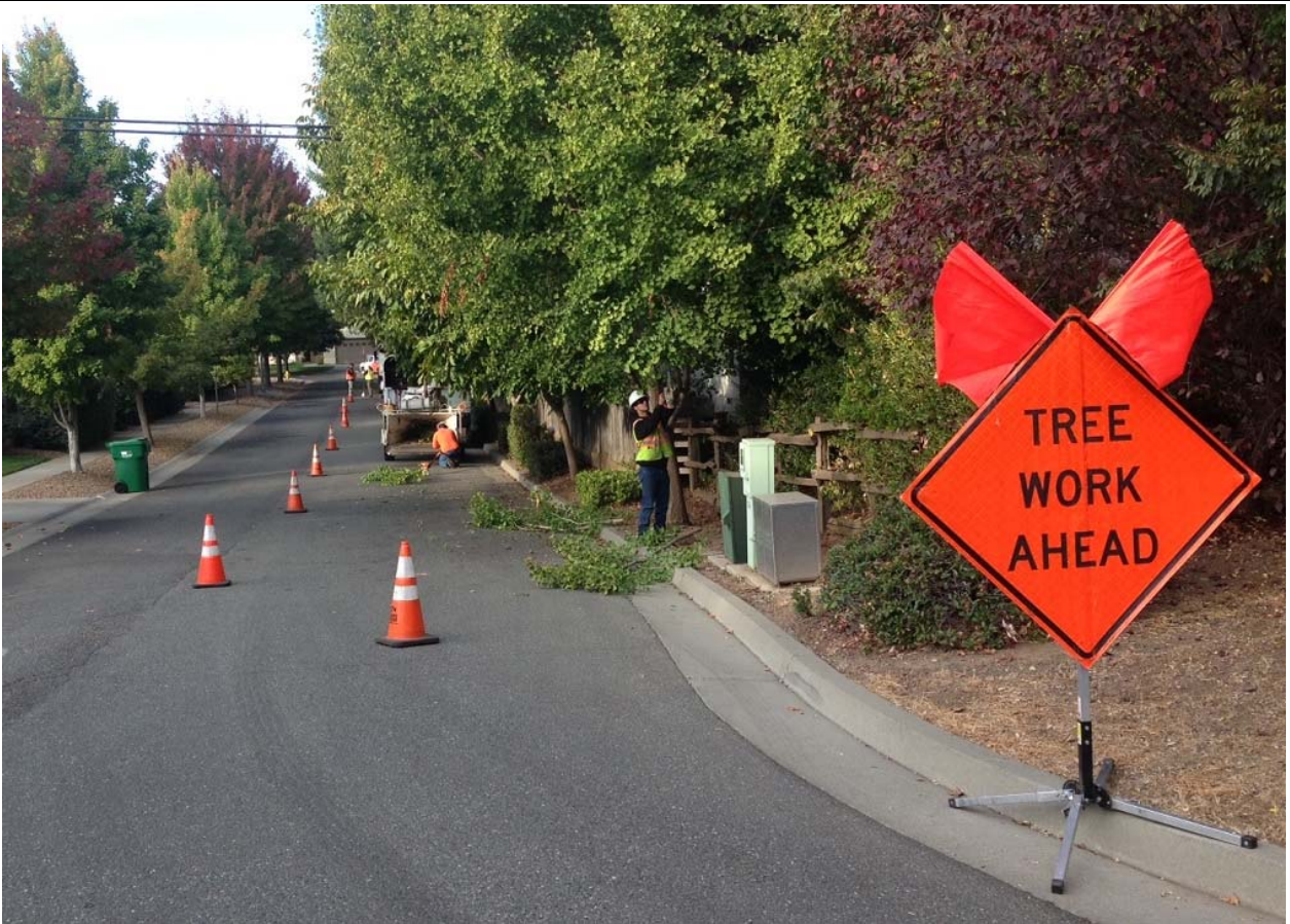
Figure 8. Public Works Tree Division on Street tree grid pruning to improve sightlines. Cosmo Dr. Tree crew pruned 996 trees
