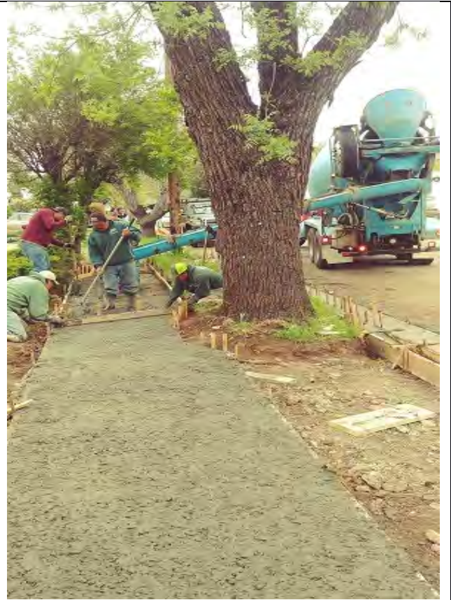
Figure 2. Developer working with UFM to save a tree in sidewalk redevelopment
