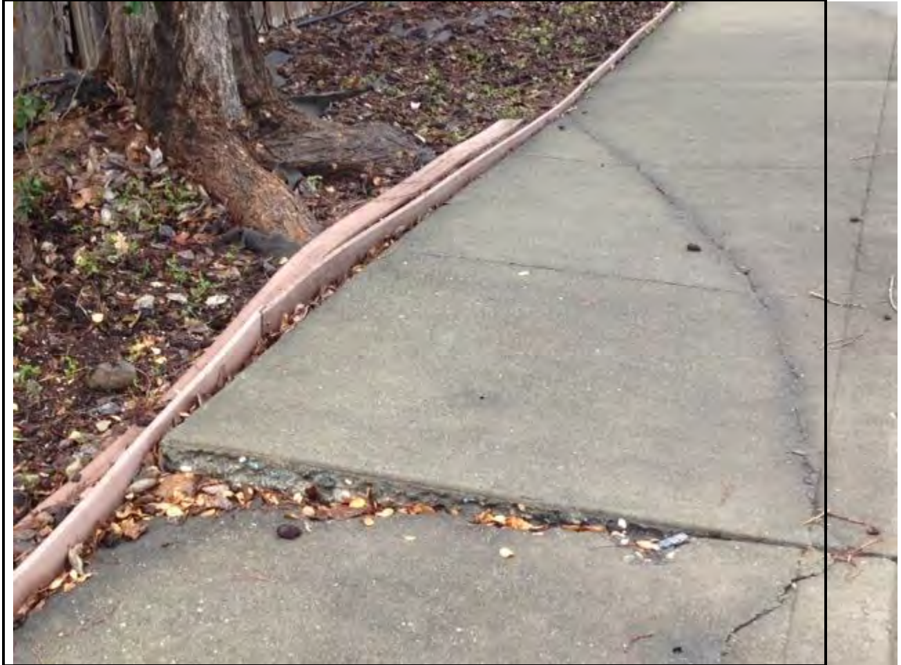
Hackberry tree next door gives a good example of what will happen in the future.
