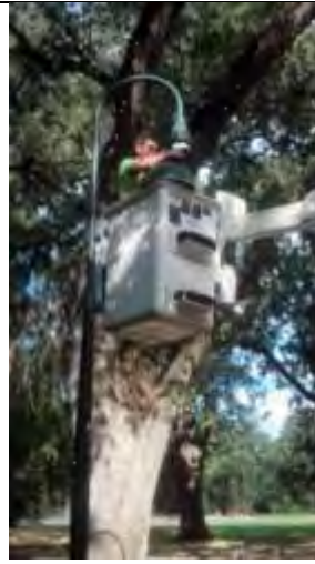
Installation of LED lights at One Mile
