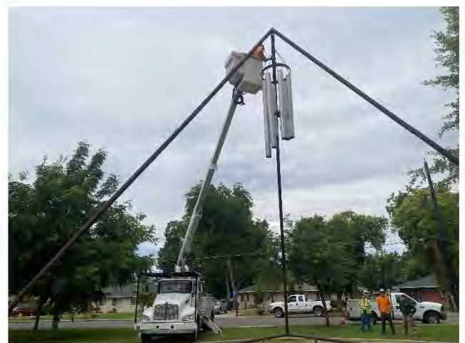
Figure 9: Tree Division and Parks staff: Windchime park
