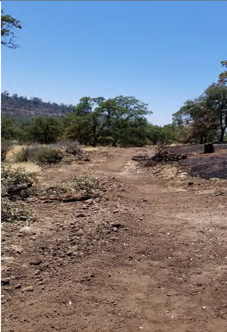
Figure 3-Middle Trail Work After Fire
