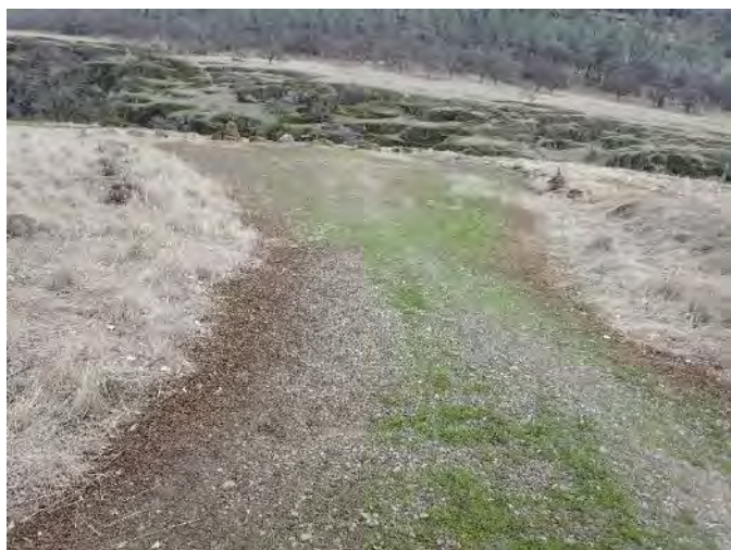
Figure 4. Each individual parking areas showed minimal signs of erosion or sediment delivery. It will important to reduce any potential run-on that may negatively affect these parking areas.
