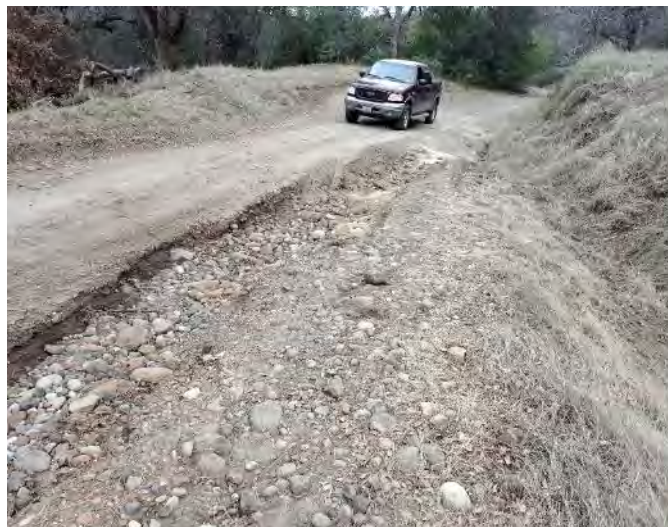
Figure 3. Vehicular passage with a 2wd car is inhibited by this large gully down the center of Upper Park Road.
