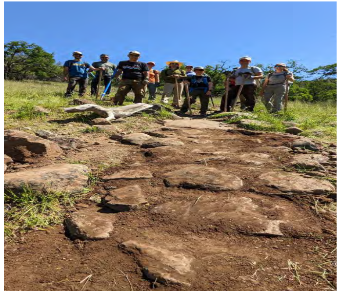
Figure 4 Trail armoring Trailworks Volunteers
