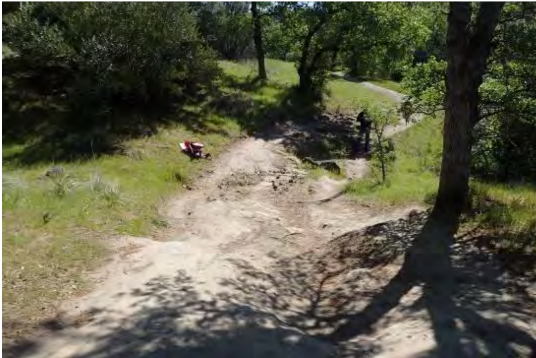
Photo 3. View of Lower Trail and PWA Geologist standing in the shade in the background. Multiple trail paths increase the trail width and this increases the area of bare soil and potential surface erosion and volume of chronic sediment delivery that will occur during storms.
